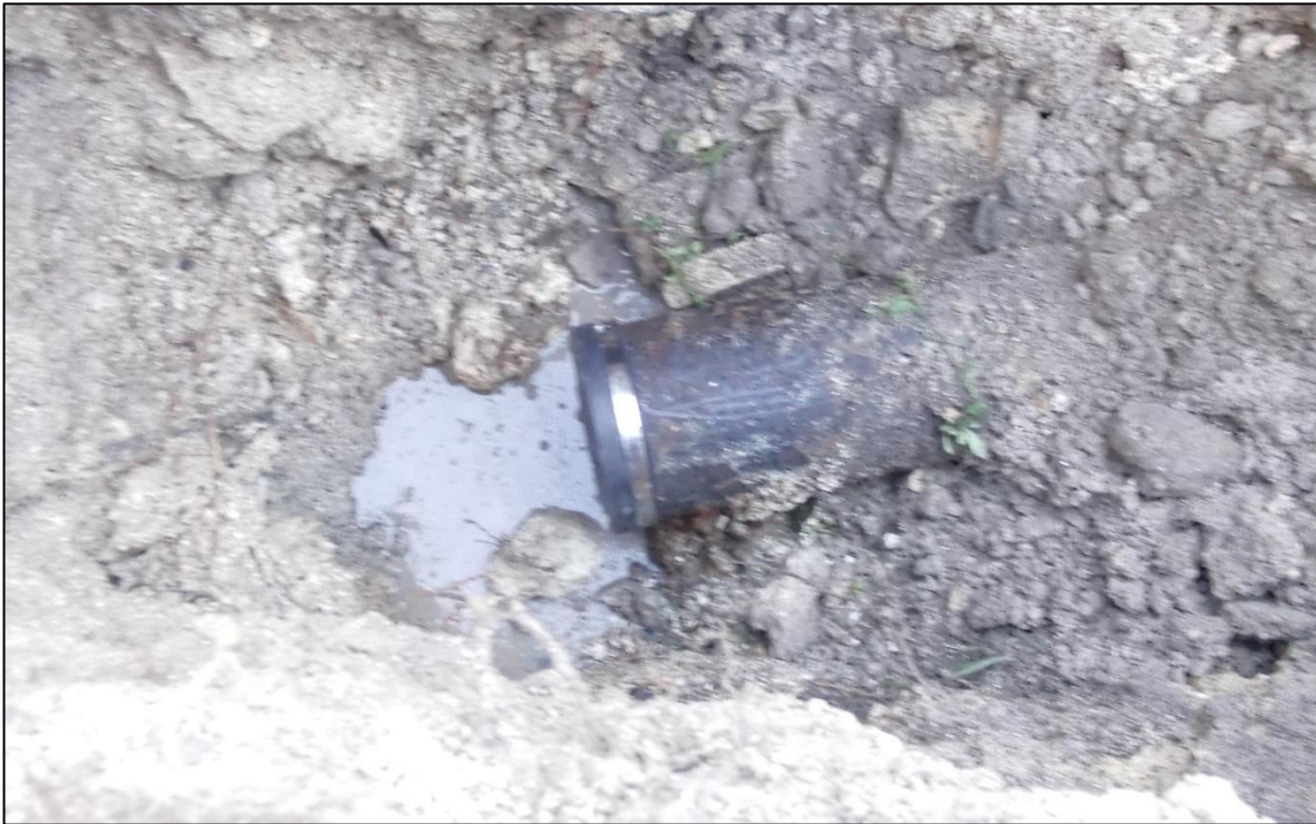
Figure 3-3: Repair of Lateral between MH 5 – MH 4
