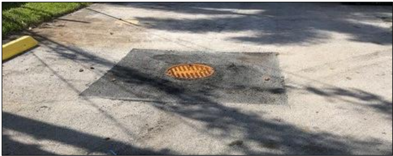
Figure 3-4: MH 100-6-2 Completed Repair
