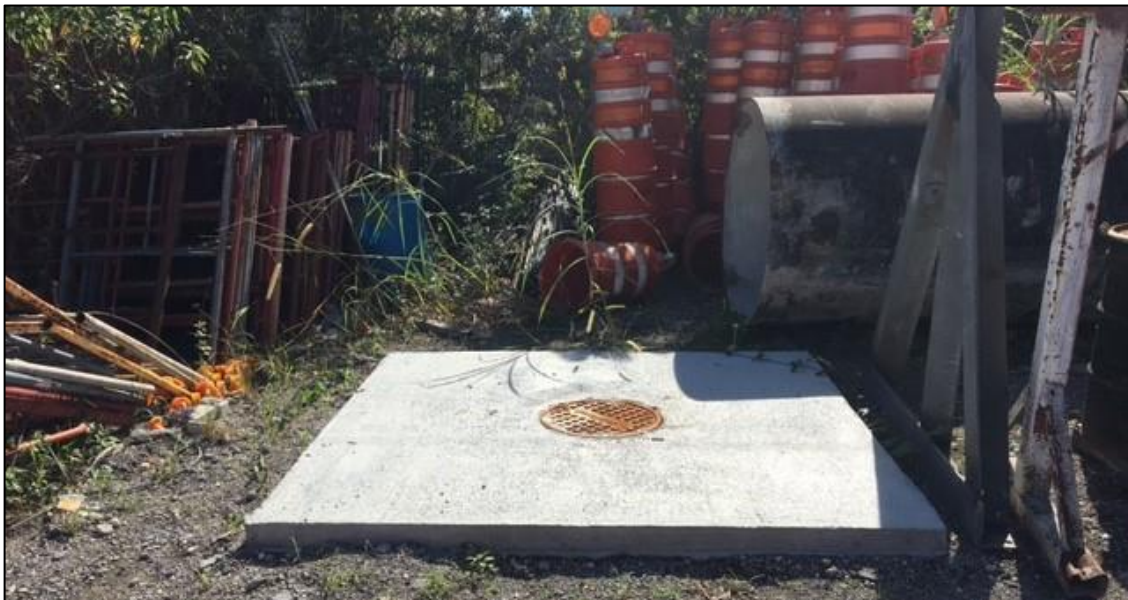
Figure 3-1: MH 9 Completed Repair
