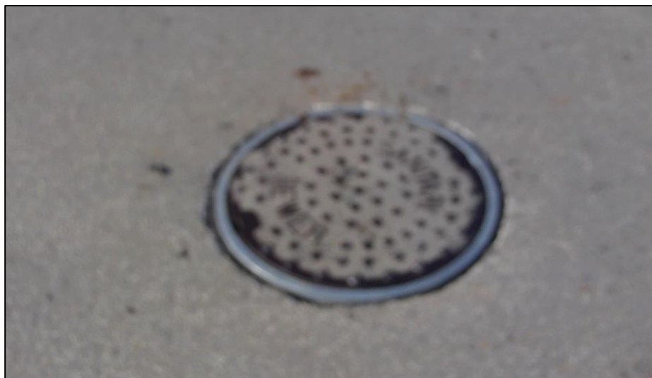
Figure 3-5: MH 103-5 Completed Repair
